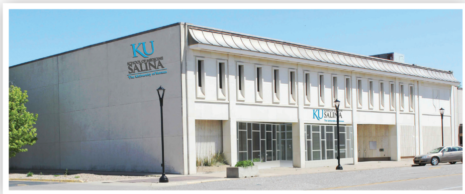
Interior demolition of the former bank building at 138 N. Santa Fe Ave, is nearly complete. New construction inside the facility will soon be underway. This image depicts future signage for the new home of the KU School of Medicine scheduled to open in 2018.
